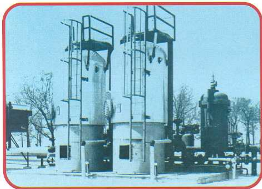
Typical BS&B LPG Dryer. This unit has a capacity of 1600 GPM
